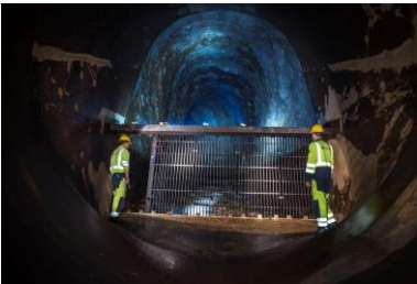
Trash rack in the Duge power plant
