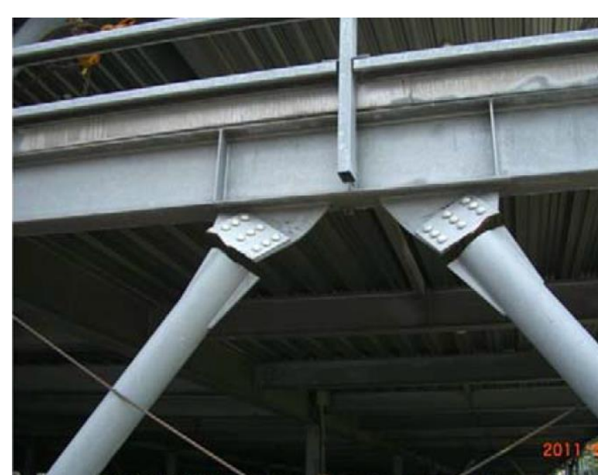
Fig. 2: Fractured Gusset Plates
